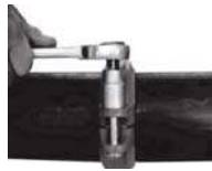
6. Tighten nuts
