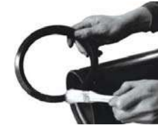
2. Lubricate gasket
