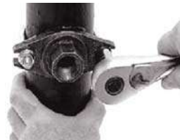
5. Tighten nuts
