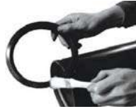
2. Lubricate gasket
